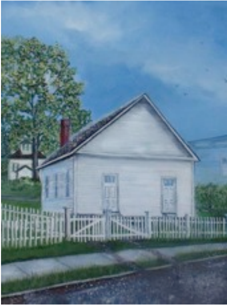
First United Methodist Church Ticonderoga, NY Built 1870
